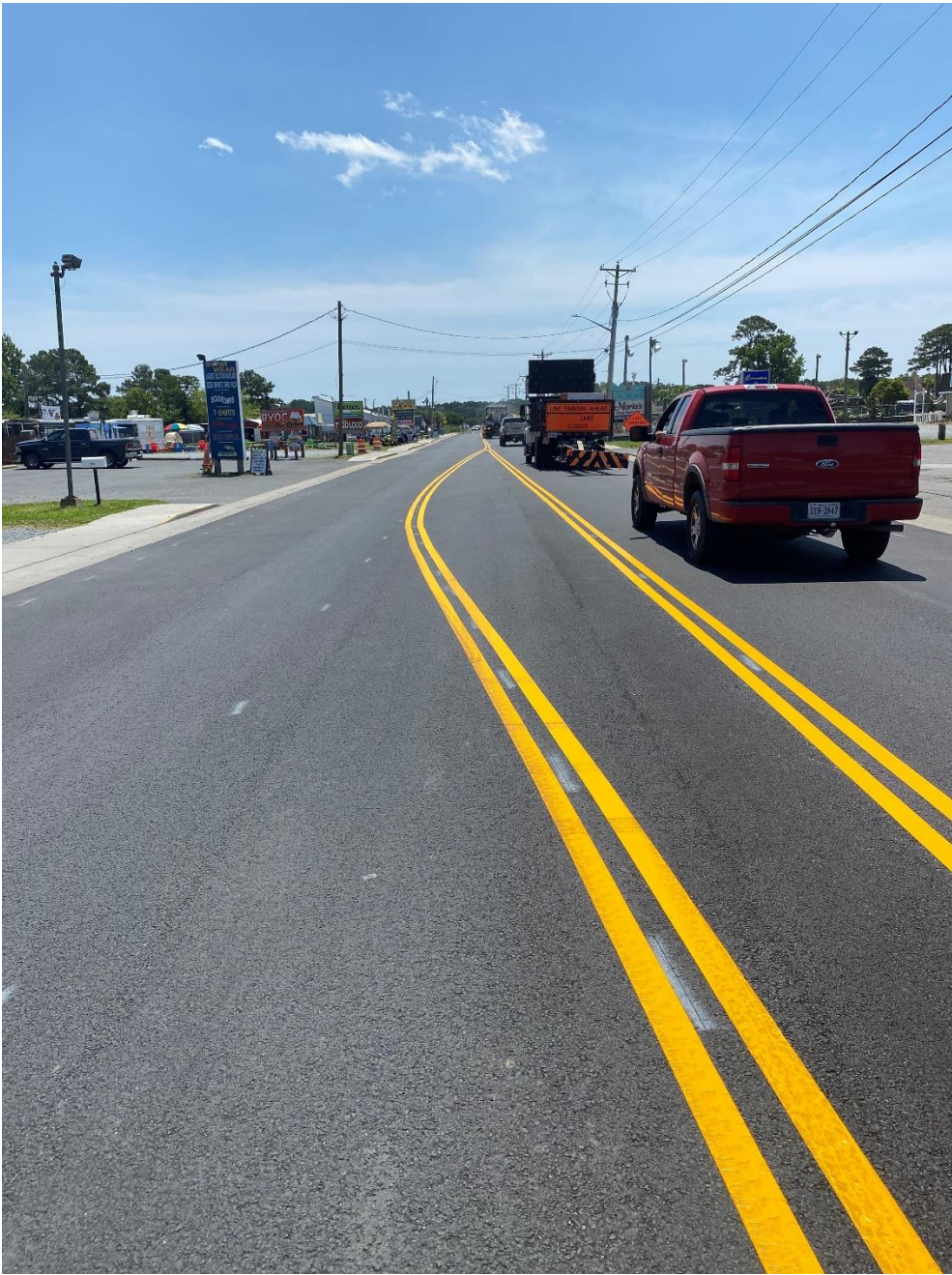
Maddox Blvd. completed including pavement markings
